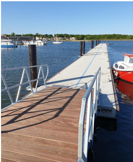
Nykøbing Mors – Beton Flydebro
